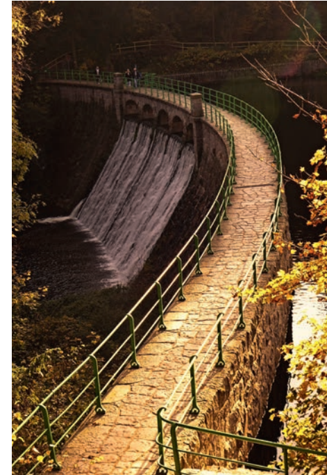
Dam at the Łomnica River
